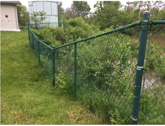
Back Fence of Plant
