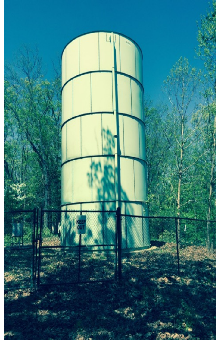
Main Standpipe (storage tank) located off Lewis Road near new entrance (holds 100,000 gallons).
